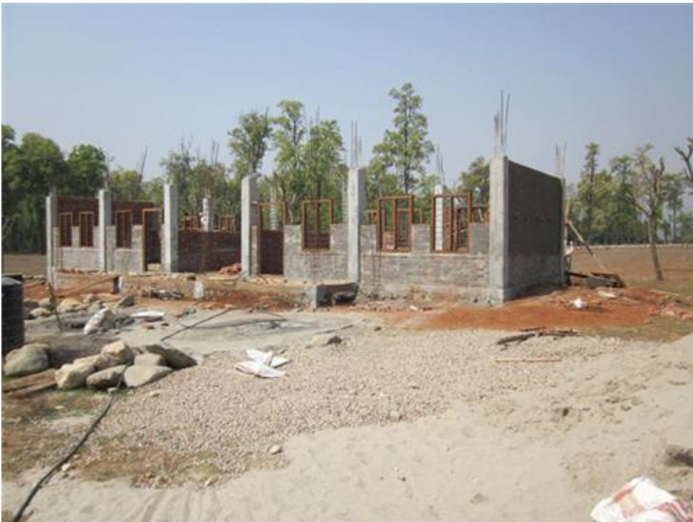
Construction work of ground floor.
