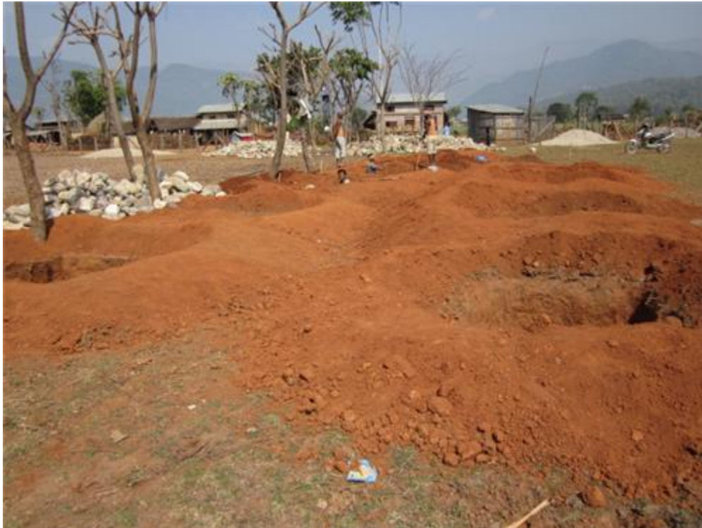
Excavation of trench.
